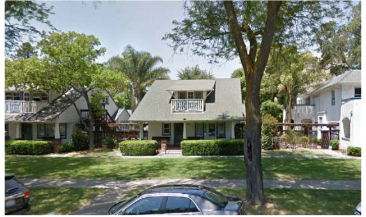
View north on First Street - Bryson House
